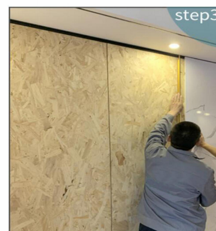
3. Install the aluminum accessories on the seams.
