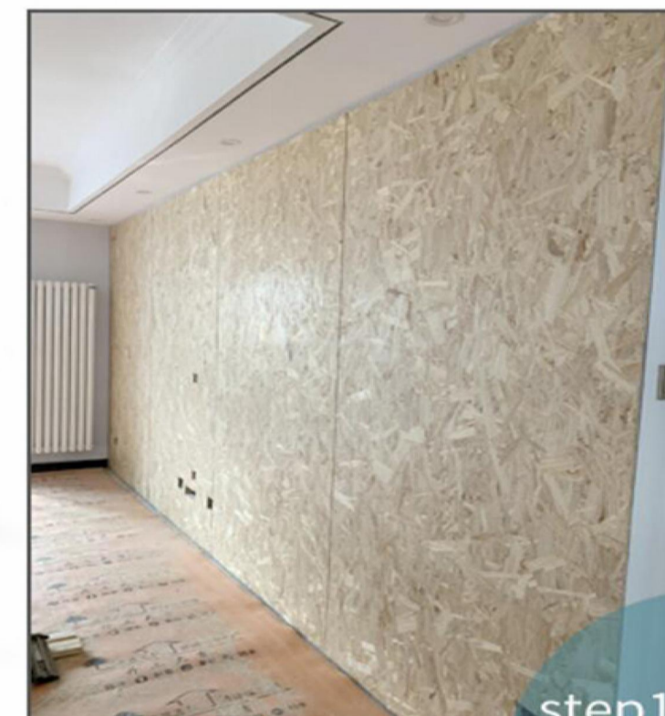
1. Make the wall base in same level
