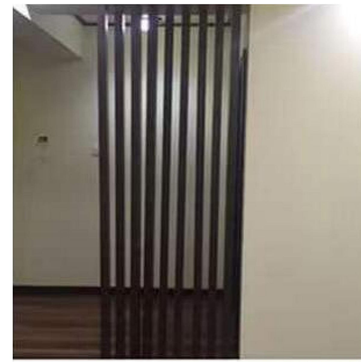
4. Finishing Timber Installation.
