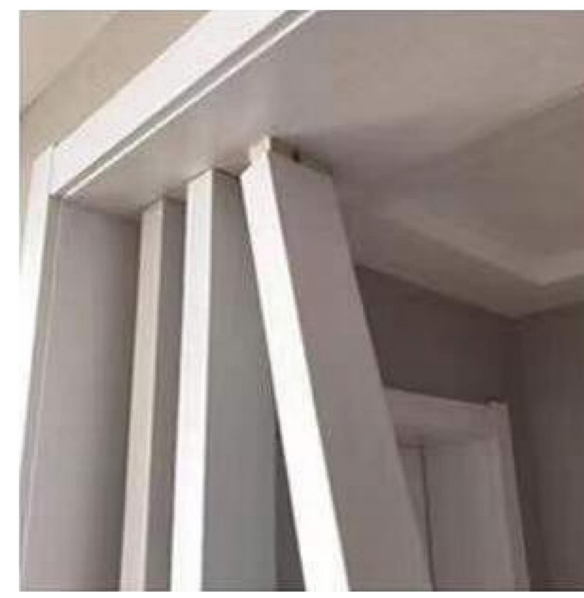
3. Fixing the timber and wood blocks on the top.
