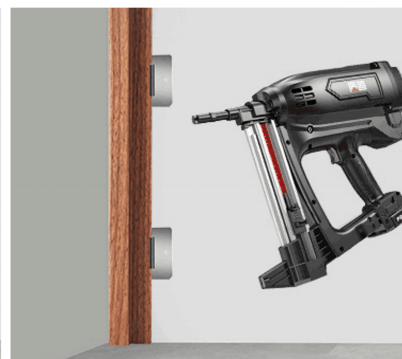
Step 2: Snap the clips into panels and then fix the clips with screws on wall by using electric drill.
