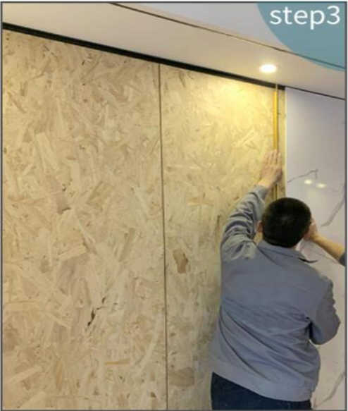
3. Install the aluminum accessories on the seams.
