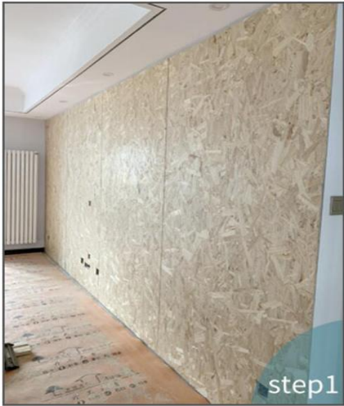
1. Make the wall base in same level.
