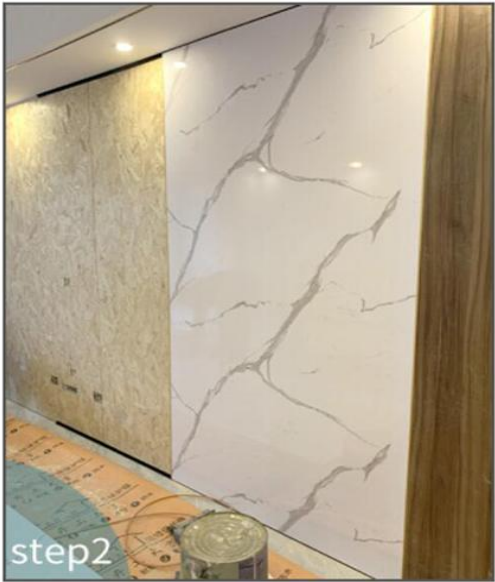
2. Put adhesives on the back of WPC wall sheet and then install WPC wall sheet on the wall.
